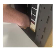
3. Use nut to secure screw from inside mast with other hand (as shown).
